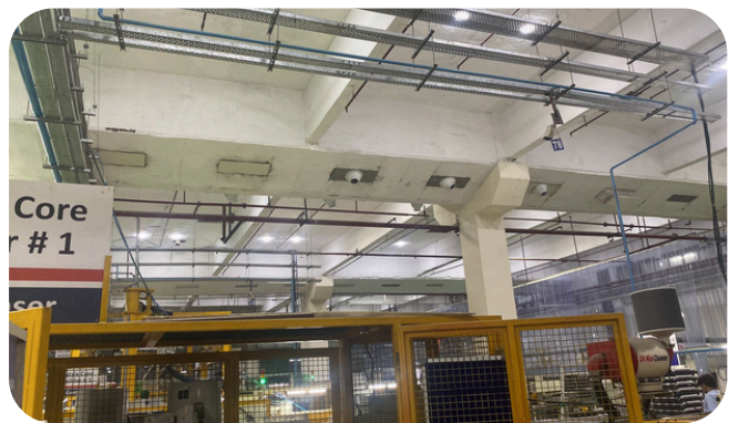
DUCTING AND STRUCTURE WORK
