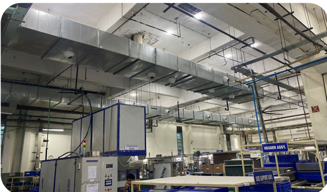
AIR WASHER DUCTING INSTALLATION WORK
