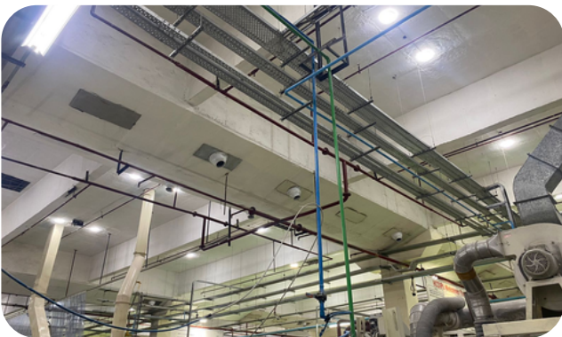
AIR & FIRE LINE WORK
